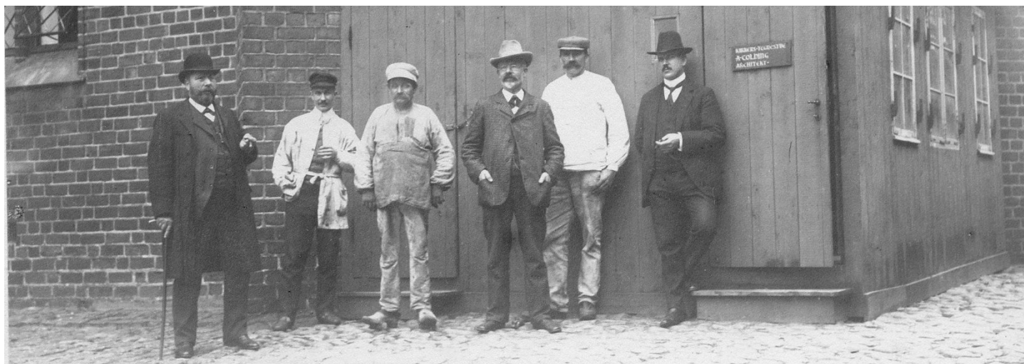
Nyborg Kirke, restaurering ca. 1870 – 1982.
